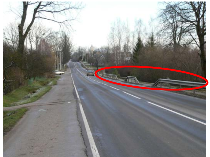
Fig. 4. Protective guardrails erected at the pedestrian-bicycle track running through the settlement
