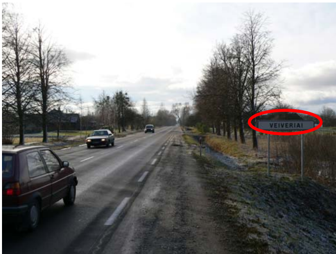
Fig. 3. The beginning of Veiveriai settlement. Having entered the settlement the road parameters do not change
